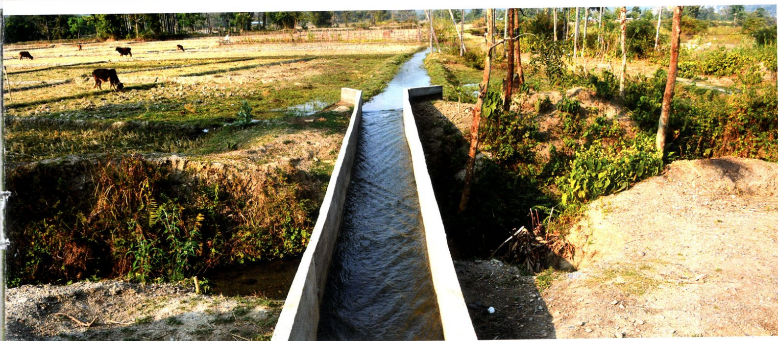
A concretized Naodara, unavoidable part of the community's water management at Nagrijuli.
